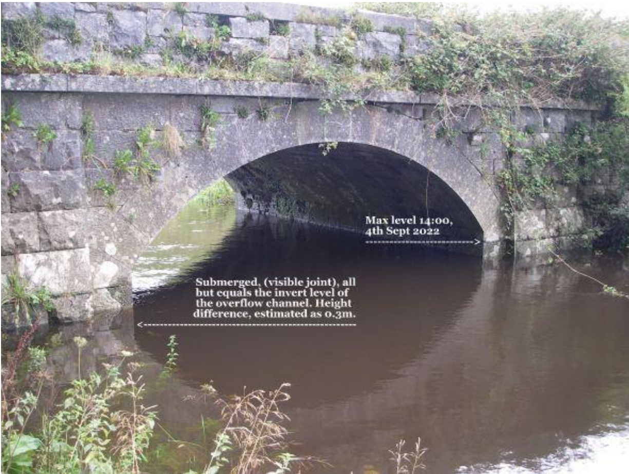
View southeast, of water levels in relation to invert of overflow channel adjacent F3a.
