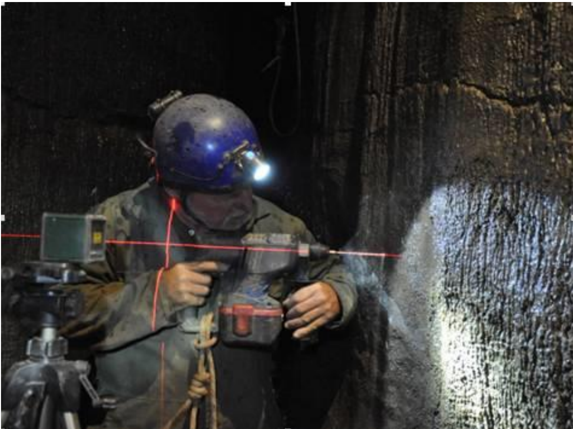
Installing staging stemple anchors at -14.6m:
