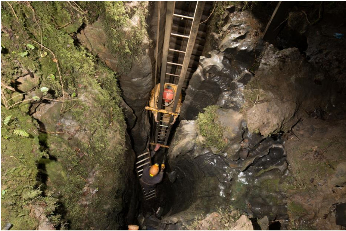
Considine's Cave installing second fixed ladder, to also act as a brattice Left to right Cheg and Pat
