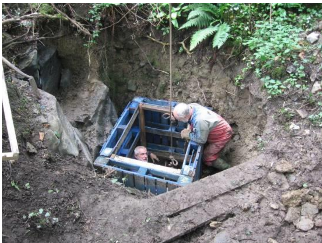
Poulfaicaislean: Pat securing shoring with Toe overseeing work.
